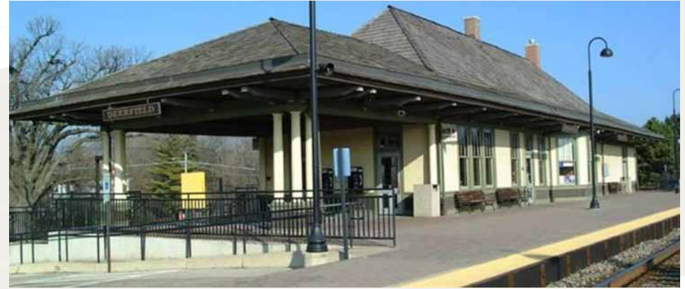
Deerfield Metra Station, Historic Renovation
